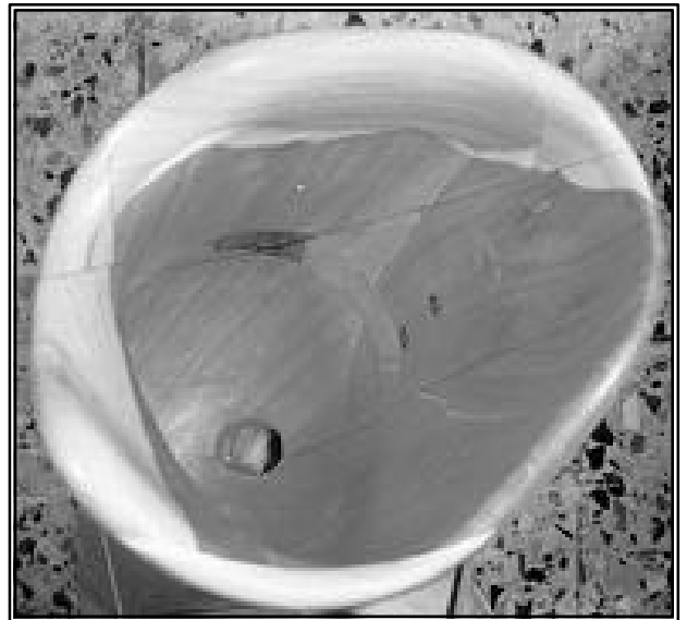
Example of a socket deepened by the affixing of a washer, tightened by a saw kerf and corrected by the insertion of additional pieces of wood.
